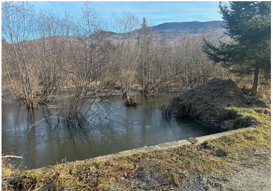
A culvert plugged with beaver debris.
