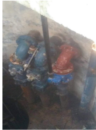
The pump station (left) with a retrofitted valve handle (right) allows for safer operation from ground level.
