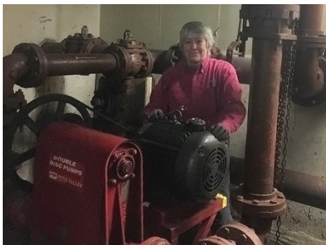
Elizabeth Walker installing the pump.
