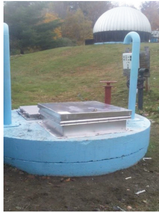
The pump station (left) with a retrofitted valve handle (right) allows for safer operation from ground level.
