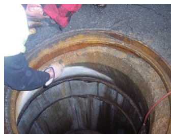
Left: sand shows the path of water. Right: deteriorating concrete under the manhole cover.
