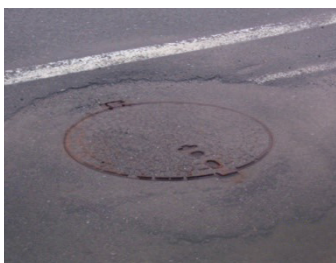
Left: sand shows the path of water. Right: deteriorating concrete under the manhole cover.
