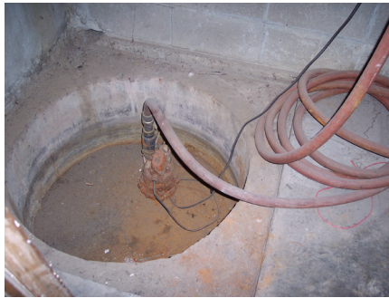
Left: a typical sump pump in a basement. Right: an illegally connected sump pump, hooked to a building's sewer line that flows to the municipal wastewater collection system.
