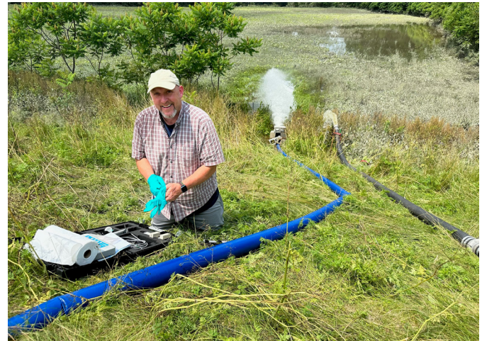
Paul Sestito setting up a bypass pump in Waterbury.
