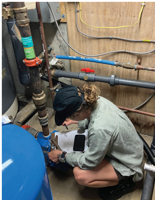
DWGPD staff performing a service line inspection at an NTNC school. Photo provided by DWGPD.
