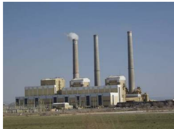
Figure 31. Coal-fired electric power plant.
