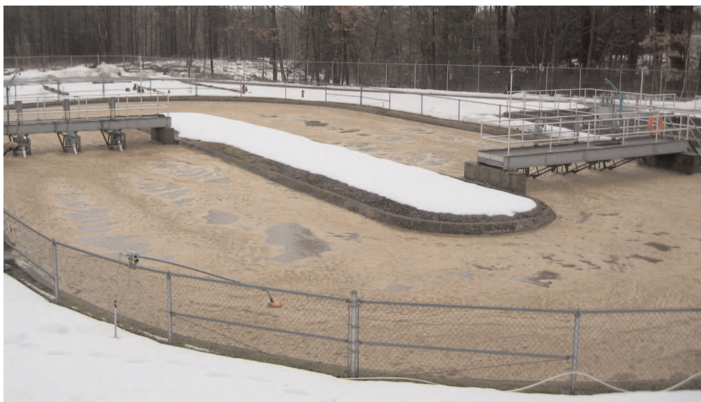
The ditch at the Fair Haven wastewater plant.
