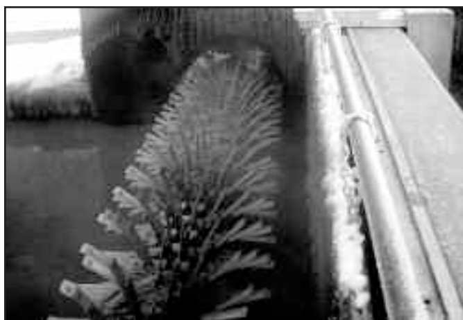
The catwalk wall last year (above) and the same catwalk wall under similar temperatures with the addition of the heated splashguard (below).
